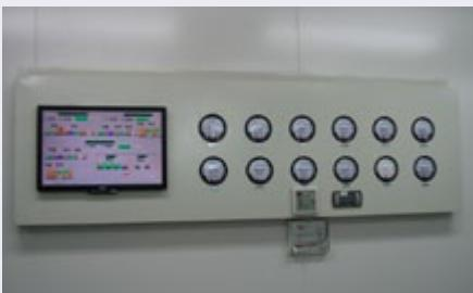
Controller of the integrated air conditioner system (2009)
