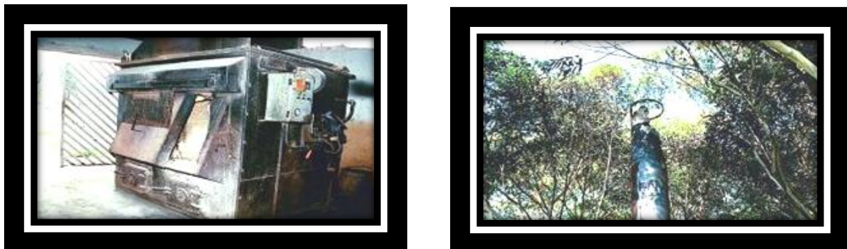
Fig 2.3.4.2: An Incinerator (l) and a Corroded Incinerator Chimney (r) (Mathunjwa 2009).
