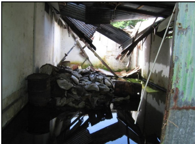
(Photo by the Ministry of LVV and John Vijgen, 2008)
