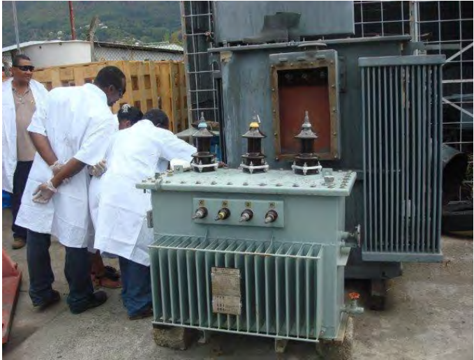
Getting access to transformer manufacture plate
