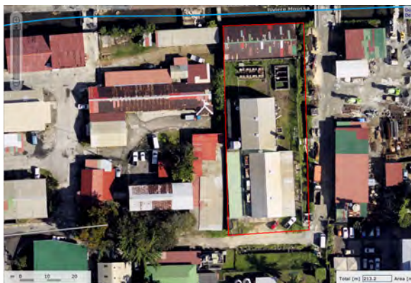
Plate 4 : Ex PUC power station at Huteau Lane on Mahe (PCB)
