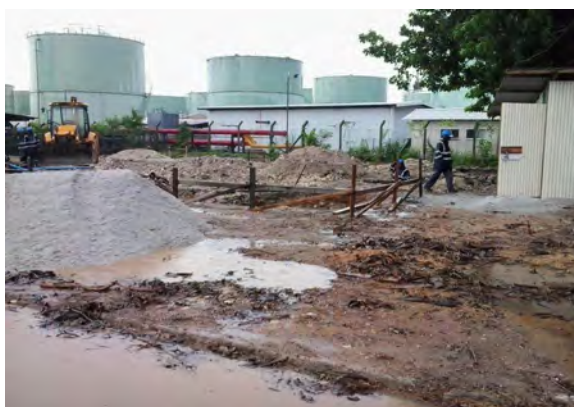
March 2014: construction of LPG distribution center in the area
