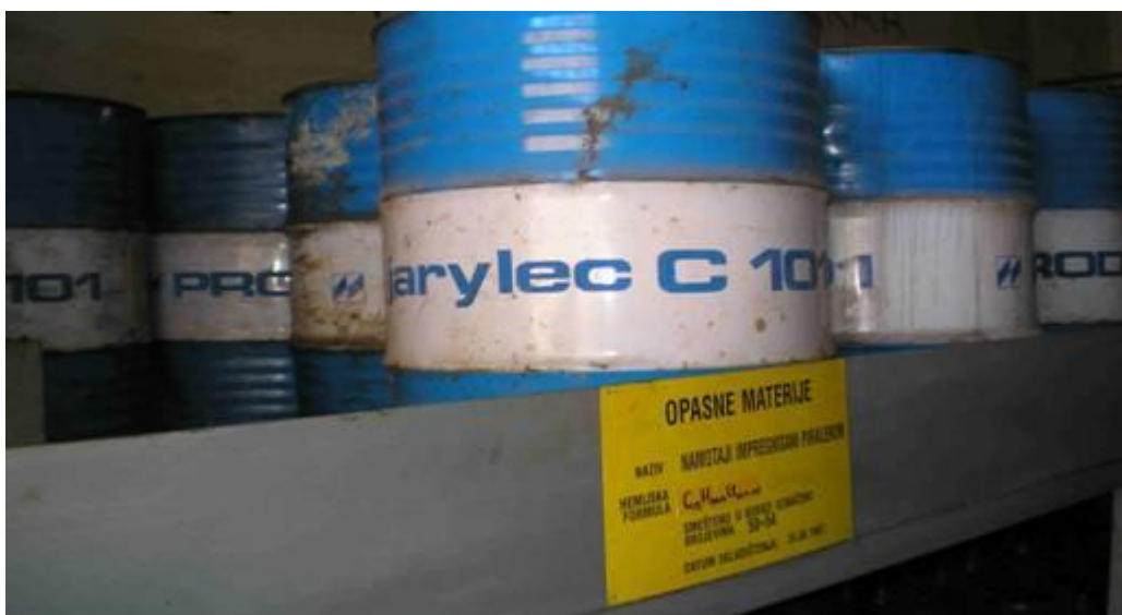
Figure 2.3.5.3.a: Stored equipment contaminated with PCB-based fluid
