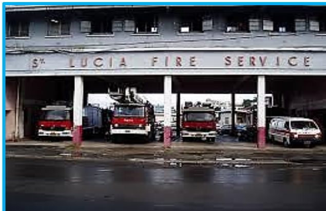
Figure 2-11: Saint Lucia Fire Services Station in Castries
