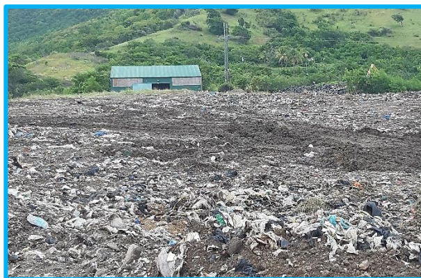
Figure 2-15: Landfill operations at the Vieux Fort Landfill Photo taken October 2019
