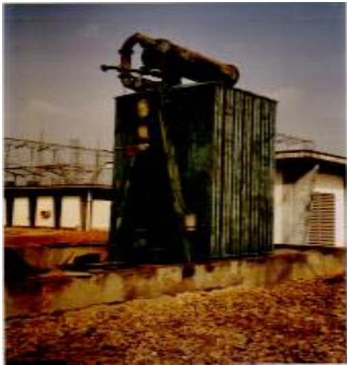
Figure 2.7 Transformer Oil spillages at transformer base in Oshogbo and oil drums stored in open air
