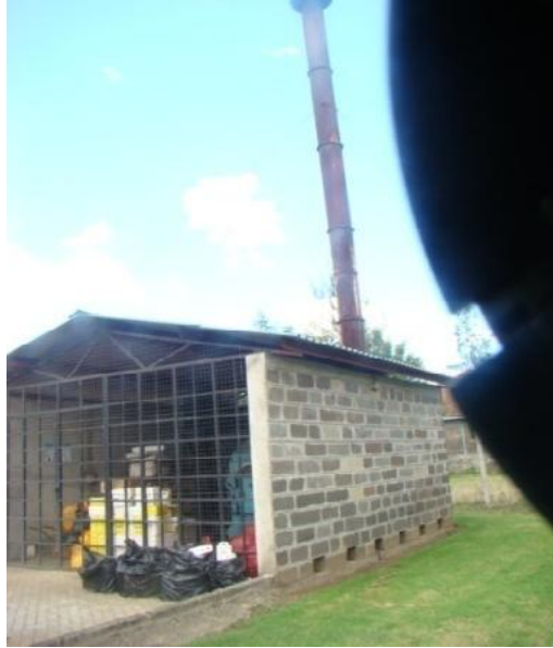
Figure 10 Nakuru Provincial Hospital Municipal Solid Waste Incineration
