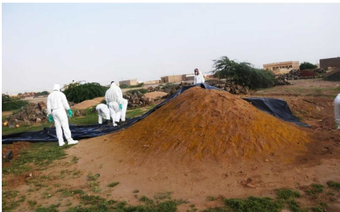
Figure 22: Temporary safeguarding activity in contaminated site at Massawa
