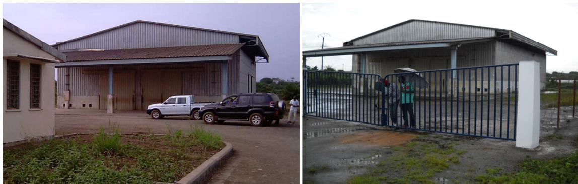
Figure 7 : (a) Warehouse KR2 in Edéa before rehabilitation (NIP, 2012) (b) after rehabilitation as Infrastructure for Temporary Storage pending their elimination
