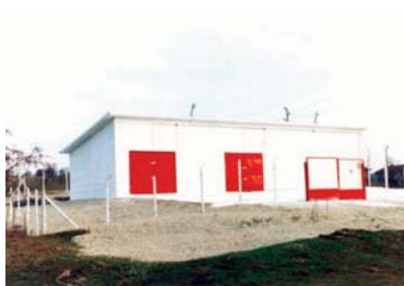
Picture 2. Repaired storage for obosolete pesticides
