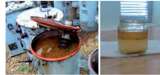
Electrical appliances with oil and water mixture
