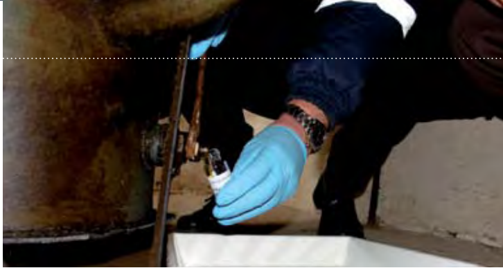
Sampling at bottom valve with drip tray under drain
