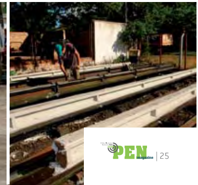
Process of concrete pole production using waste oil
