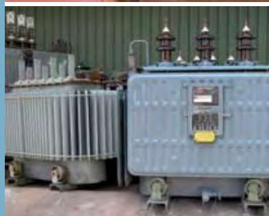
Dismantling of a PCB transformer
