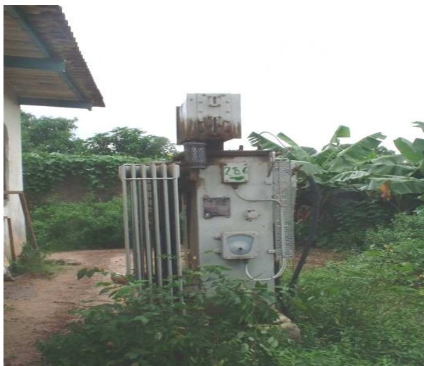
Plate 2.2: Leaking electrical transformer in an abandoned area in an African country (Source: GTZ PCB Project, The Gambia 1/6/2000)
